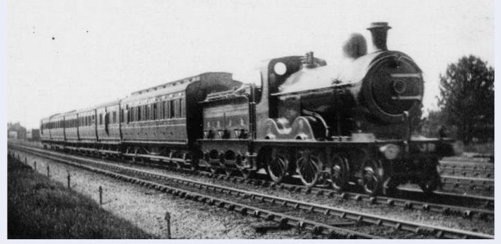
Rebuilt small Johnson 4-4-0 No.18 passes the carriage sidings on its descent towards Bournemouth West with a through passenger on Saturday 31st May 1913. No.18 was one of the four original small 4-4-0 locomotives to be built by Derby for the S&DJR, arriving in May 1891. They immediately took on the heavier passenger workings which had been previously entrusted to the thirteen 0-4-4T locomotives, subsequent Derby deliveries relegating the latter to local and branch lines
