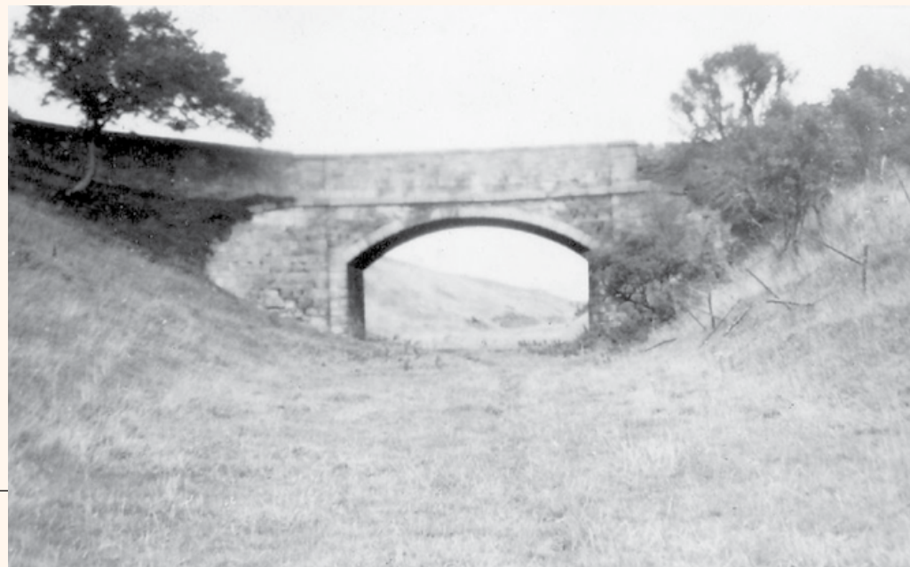
This photograph, taken in the 1920s, shows an early alignment of the ECML close to the friable sandstone cliffs. By this time the line had been realigned further inland for safety reasons and to make sure that vibrations from passing trains no longer caused the unstable cliffs to collapse. The parapets of this bridge are visible today but the railway is crossed by a new bridge closer to Marshall Meadows Farm. (The late Neil Mackichan)
