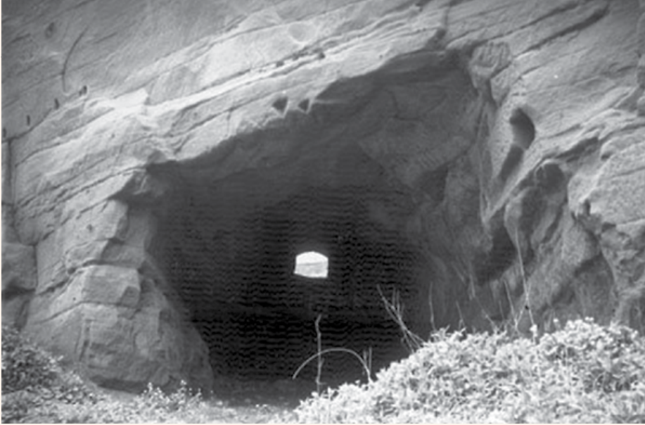
ABOVE: This view shows the late twentieth century view of the lower tunnel arch. Successive cliff collapses have caused the lower tunnel entrance to be several metres above its original position. The original stone arch over the entrance has long since disappeared.
