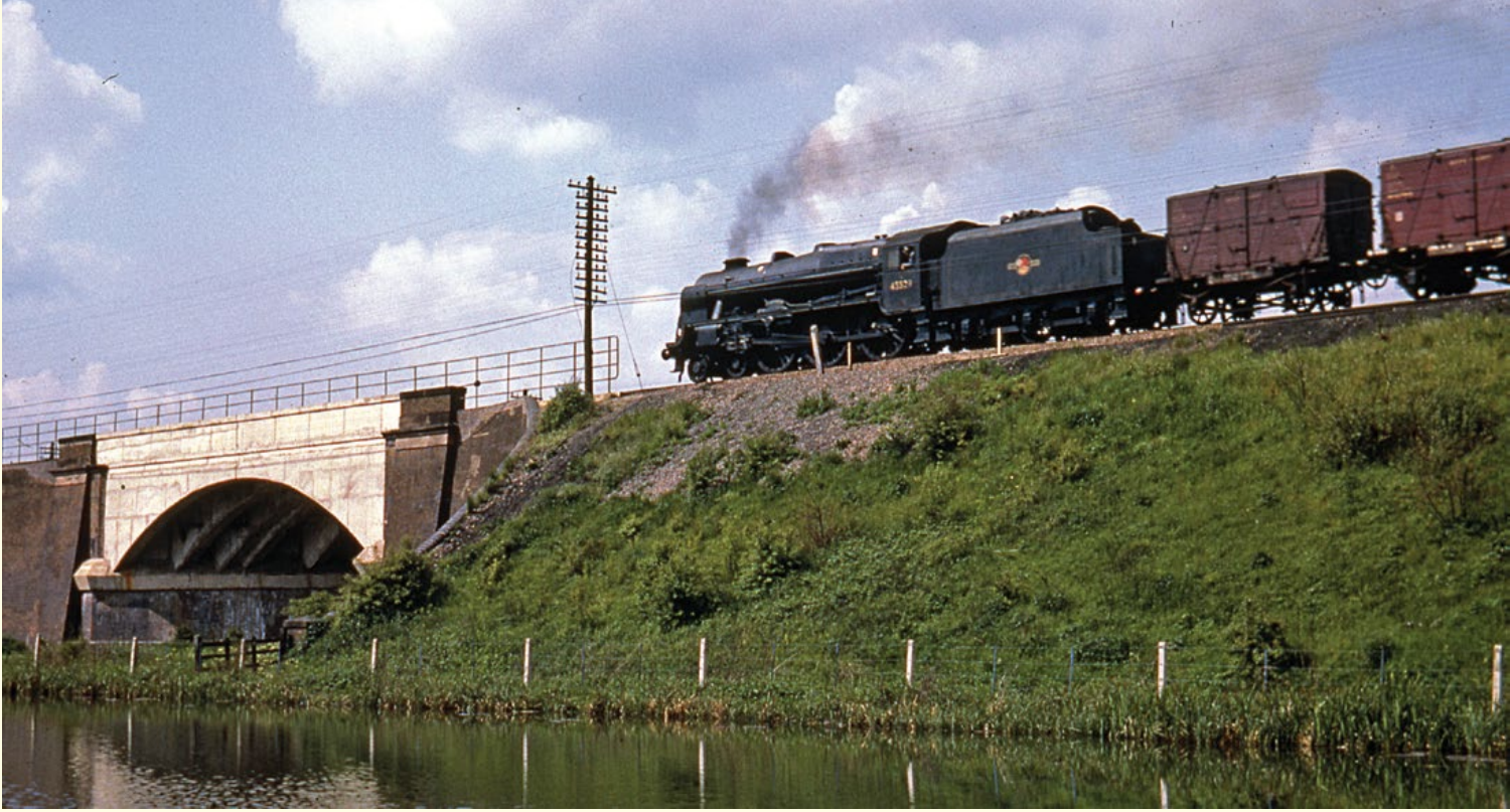
TOP: Rebuilt 'Patriot' No.45529 Stephenson is about to cross the Grand Union Canal at Apsley with a northbound express freight in 1962. Modernisation is coming to the WCML and Robert Stephenson's original skew arch has been strengthened by being encased in concrete.
