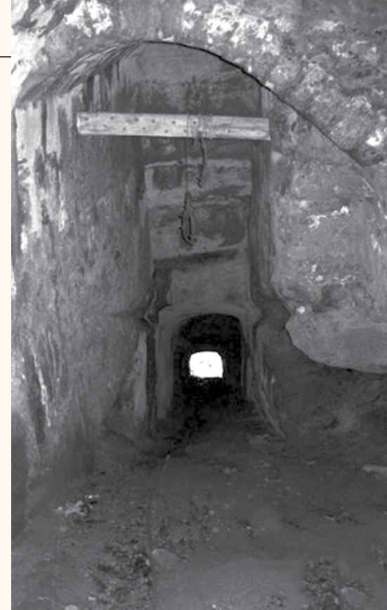
ABOVE: This view shows the late twentieth century view of the lower tunnel arch. Successive cliff collapses have caused the lower tunnel entrance to be several metres above its original position. The original stone arch over the entrance has long since disappeared.
