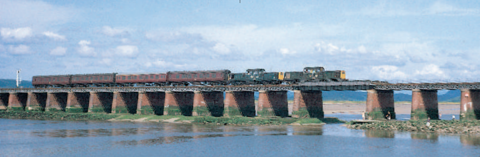
ABOVE: An engineering feature of the Furness line is the series of long viaducts carrying it across the wide estuaries of rivers running down from the Lakeland fells into the sea. At Arnside the estuary of the River Kent required a viaduct of 49 spans, 520 yards long. Originally constructed in timber, it was renewed in the 1880s and again rebuilt during World War I. Two Clayton Type 1 diesels combine their meagre resources to cope with the four coaches of a local passenger train from Barrow on 2nd August 1968. (David A. Hill)
