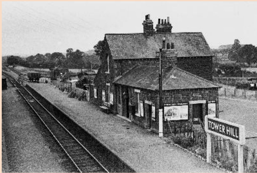
Tower Hill station in 1939. This served a rather scattered local community and was one of the least-used stations on the North Cornwall line. Note that at the time of the photograph there was only one platform line, the loop having been taken out of use just before the Grouping, though it was reinstated during World War II due to D-Day traffic needs. This is one station which has unfortunately not survived until the present day, having been demolished after closure for reasons that are not known. (Stations UK)
