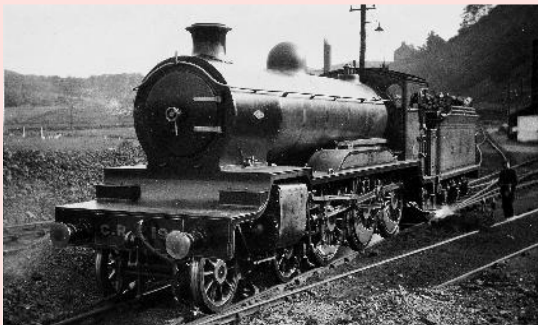
RIGHT: CR 4-6-0 No.195 at Oban shed, the third design of 'Oban Bogie', following McIntosh's Class '55' and Brittain's '179' Class. These were the last locomotives built before grouping and were delivered by the NB Locomotive Co. in December 1922. The eight locomotives were withdrawn between 1939 and 1945, a relatively short life compared with their predecessors the Class '55', the last of which was withdrawn in 1937 after 32 years of service.
