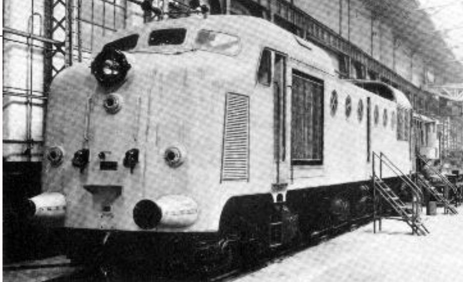
One of the Egyptian (1A) Do(A1) 1,600hp locomotives under construction at Preston. Engines for this order were transferred to the LMSR Derby Works in order to expedite the construction of Nos.10000 and 10001 and in particular No.10000 so that it could be completed before nationalisation. (EE/Author's Collection)
