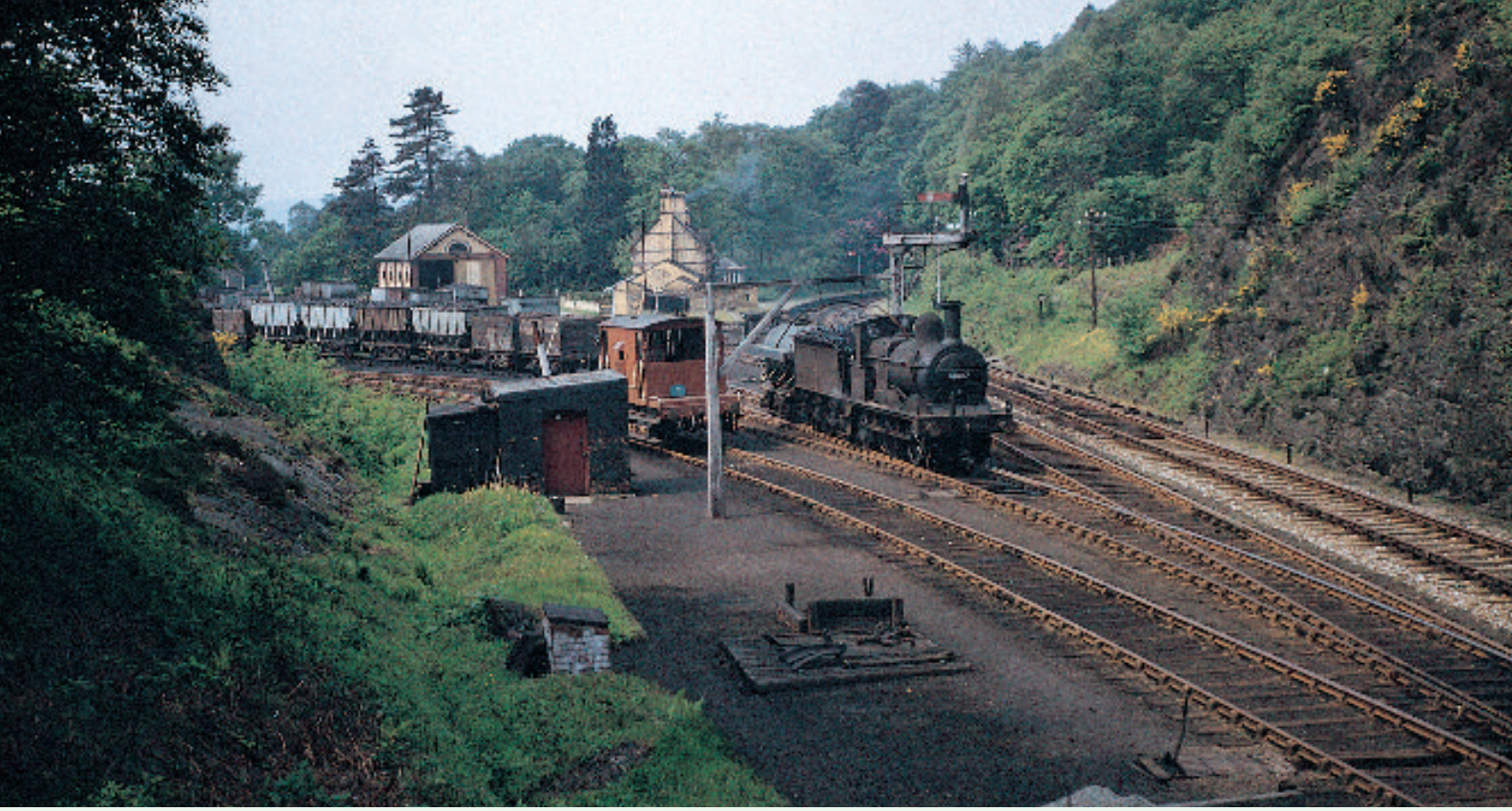
ABOVE: The branch to Lakeside (Windermere) lost its year-round service in 1938 after which (apart from a wartime interruption) it ran only in summer until 1965. Goods traffic did continue, however, and the yard at Haverthwaite seems busy on 31st May 1960 when Midland Railway 2F 0-6-0 No.58287 was shunting the sidings. The station was last used for passengers at the end of the 1946 season but was not officially closed until 1955. (J. S. Gilks)
