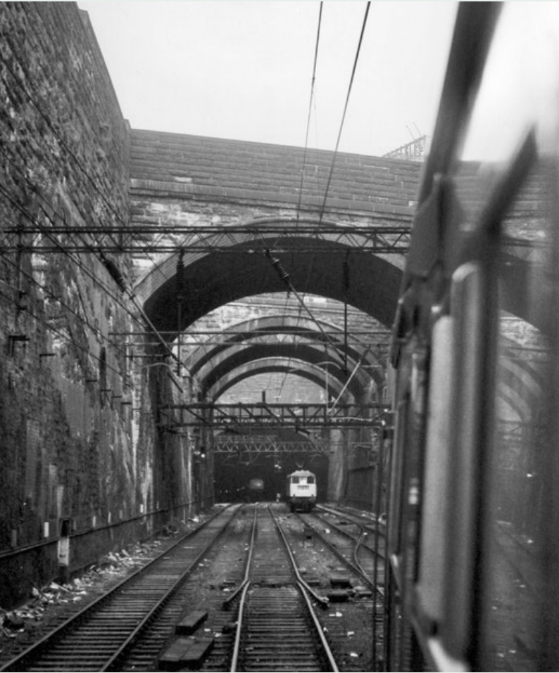
ABOVE: This is the four-track line alongside the single tunnels. The train I am on has just come from the down fast using the crossing behind and is continuing to the shunting neck. Any rolling stock leaving this without permission will doubtless be stopped in its tracks by the catch points, which are clearly designed to keep the runaway off the running lines to either side. The vent on the left, between St. Andrew and Gill Streets, appears to be the one in the last picture. The five-track span in the distance is Brownlow Street bridge, now with the other side closed in as mentioned below.
