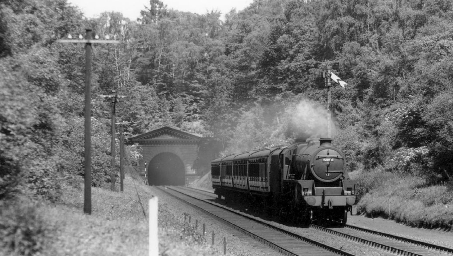
Watford Tunnel was 1 mile 70yd in length, cut through chalk with intermixtures of sand and gravel. LMS Class 5 4-6-0 No.5350 leaves it behind with a lightweight four-coach express in the late 1930s. (Pendragon Collection)
