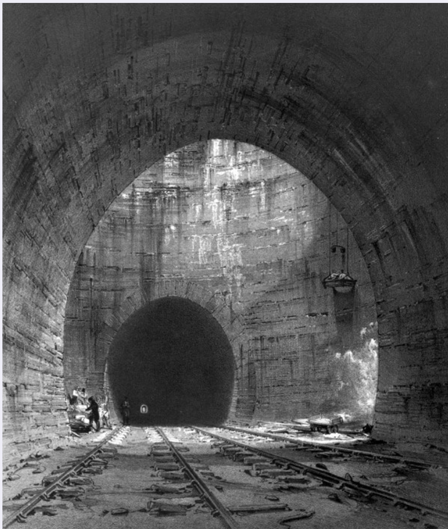
Peter Lecount’s description of Kilsby Tunnel includes a reference to the Great Shaft, which had been commenced in May 1836, taking twelve months to complete. “This shaft is sixty feet in diameter, and 132 feet deep; the walls are perpendicular and three feet thick throughout, the bricks being laid in Roman cement.” In this image, the walls and the shaft remain to be bricked. Bourne’s engraving is of one of the main shafts and illustrates that he had the temerity to walk through the tunnel ere it was completed.
