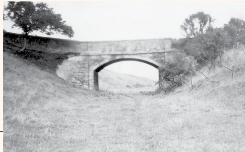
This photograph, taken in the 1920s, shows an early alignment of the ECML close to the friable sandstone cliffs. By this time the line had been realigned further inland for safety reasons and to make sure that vibrations from passing trains no longer caused the unstable cliffs to collapse. The parapets of this bridge are visible today but the railway is crossed by a new bridge closer to Marshall Meadows Farm. (The late Neil Mackichan)
