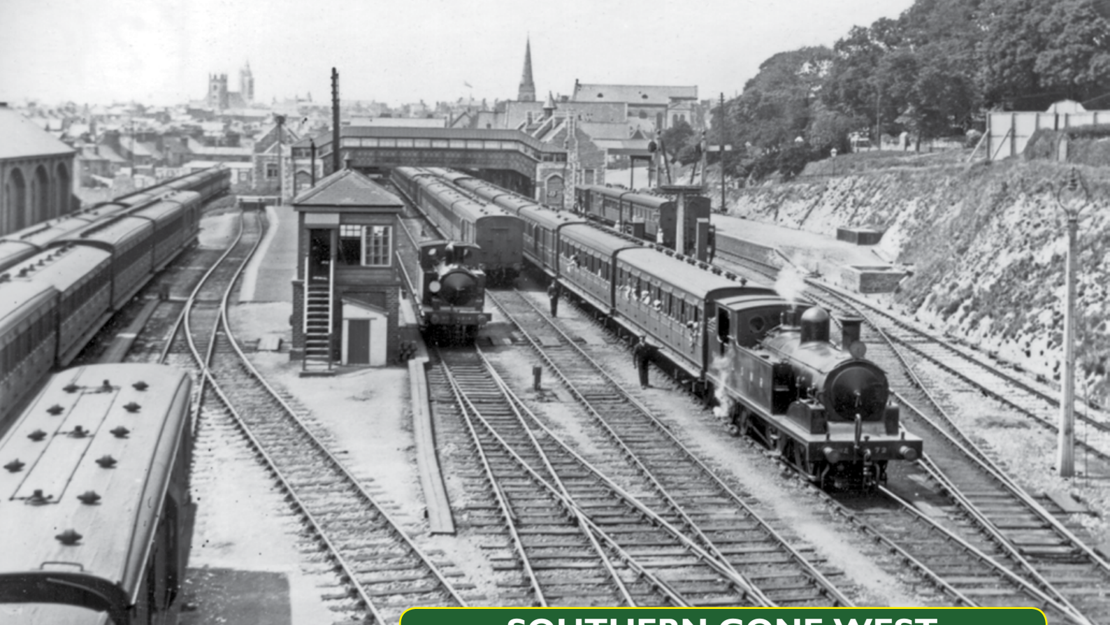
A general view of Friary station, looking west towards the buffers, on 8th July 1924 from Tothill Road overbridge. No fewer than five sidings are occupied by empty coaching stock. Adams T1 Class 0-4-4 tank departs on the lengthy 1.54pm run to Tavistock via North Road, whilst later Adams O2 No.218 waits by the Friary 'B' signal box. The O2 was to end its days as No.W33 Bembridge on the Isle of Wight, surviving until December 1966 but sadly not being preserved. (H. C. Casserley)
